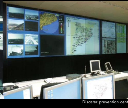
Police command & control room
